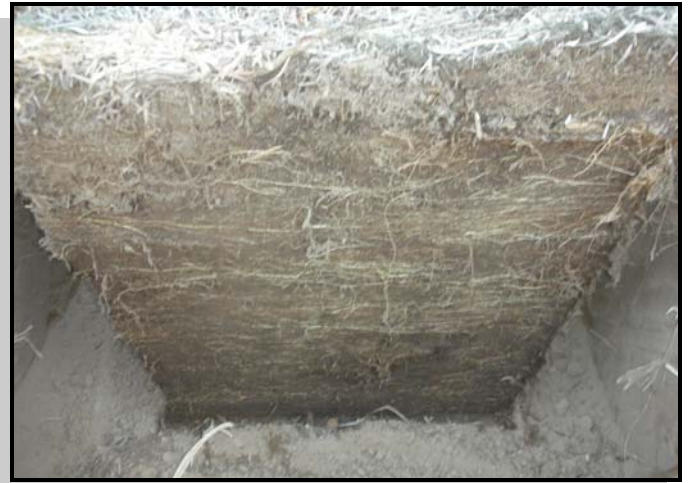
Here is a 24" box tree in the planting hole. It is recommended to shave 1/8-1/4 inch off the edges of the rootball sides to accelerate root development into the native soil.
