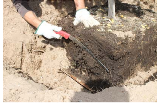
Figure 7A. For well rooted container grown trees and prior years field dug trees prune away 1/4 to 3/4" of the outer edge of the rootball removing any matted, kinked and circling roots.
