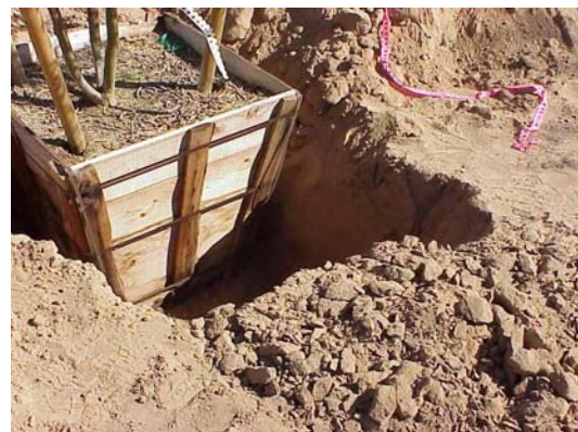
Figure 5. Fractured soil improves water pene-
